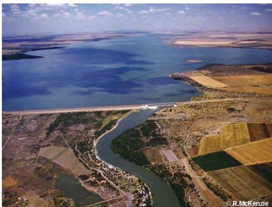
Photo 8.1.1 Bloemhof Dam: An example of the large surface area of a relatively shallow dam experiencing high evaporative losses (Photo: R. McKenzie)
