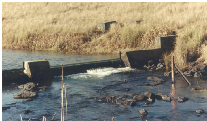
Photo 1 Illustration of a streamflow gauging structure on the Mvoti river in KwaZulu-Natal, data from which have been used in streamflow verification studies (Photo: R.E. Schulze)
